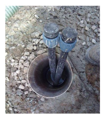
Geology impacts installation depth, drilling method, drilling costs and borehole thermal performance Contain U-tubes of polyethylene pipe Some systems utilise concentric pipes Typically installed to depths of up to 250m but may be >500m
